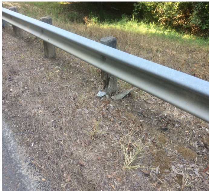
PHOTO 1 Description Guardrail post damage.
